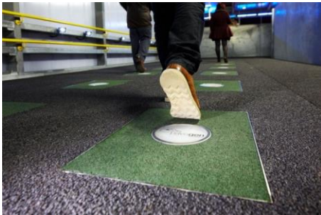
Figure 5: Tile generating energy from pressure[]
